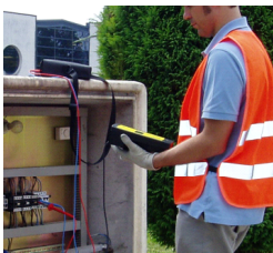
Signal injection in a power-box using the IC1G transmitter (TX)
